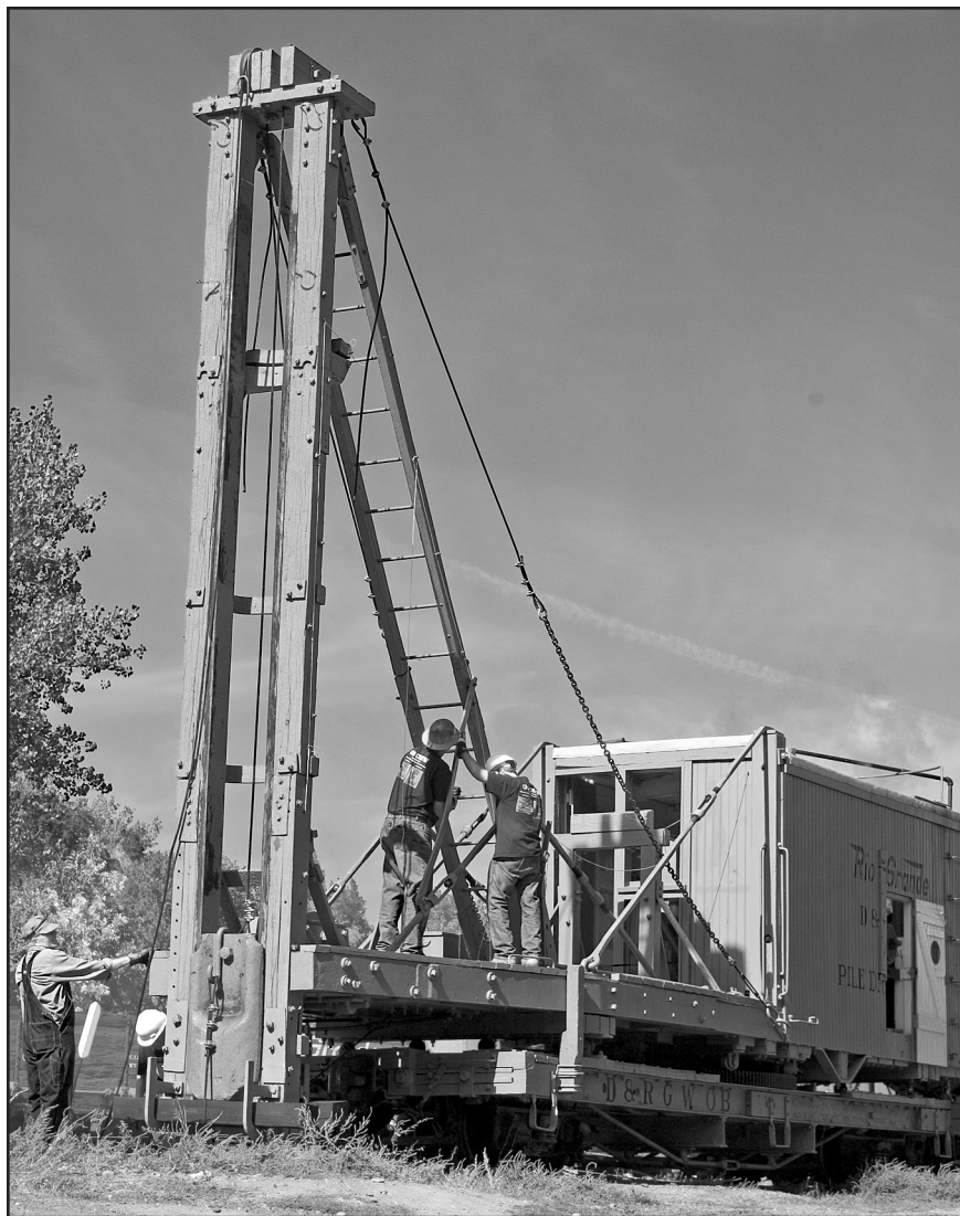
Pile Driver OB operates at the Colorado Railroad Museum on September 17, 2009. – Photo © 2009 Bruce Nall.
